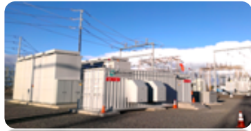
Distribution Level Energy Storage
