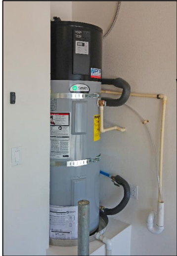
Electric Heating and Water Heating
