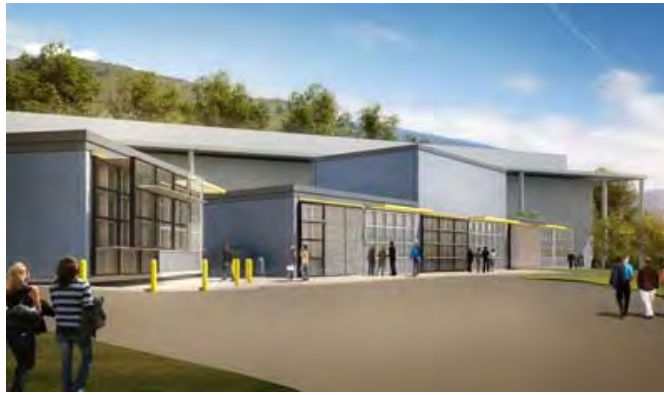
The new, exterior portion of FLEXLAB will host four new testbeds.
