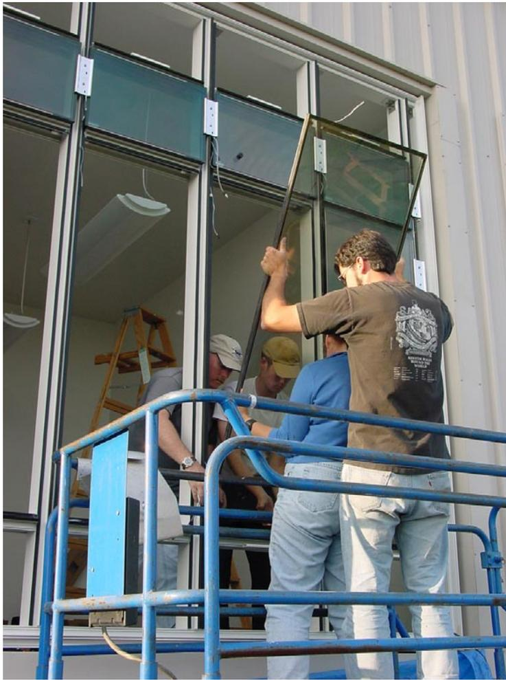
Figure 2. Installing windows
