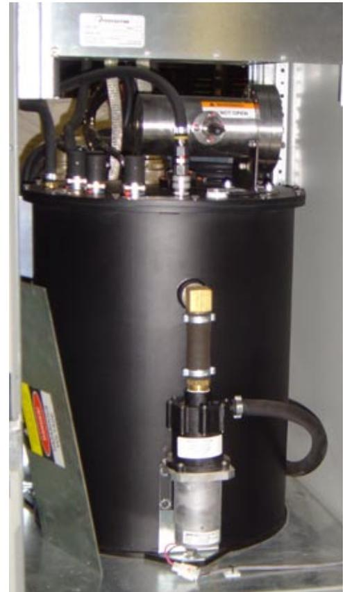
Figure 1. Flywheel uninterruptible power supply (UPS)
