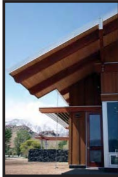
Figure 1. The design team included light-shelves and sun shades, highly reflective roofing, and fenestration that minimizes heat gain and loss and maximizes views of Mt. Whitney. (Photo: Bill Hustace)
