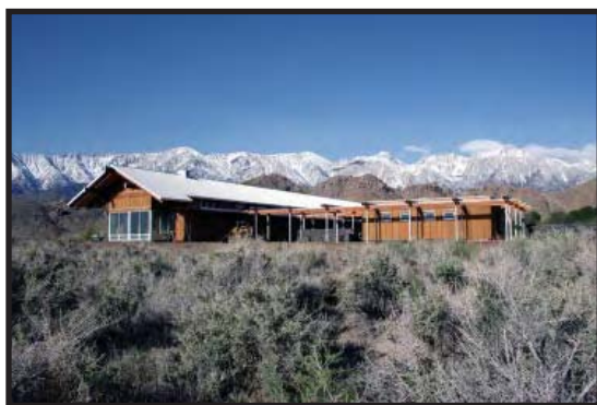
Figure 2. The Eastern Sierra Inter-Agency Visitors Center, Lone Pine, California (Photo: Bill Hustace)
