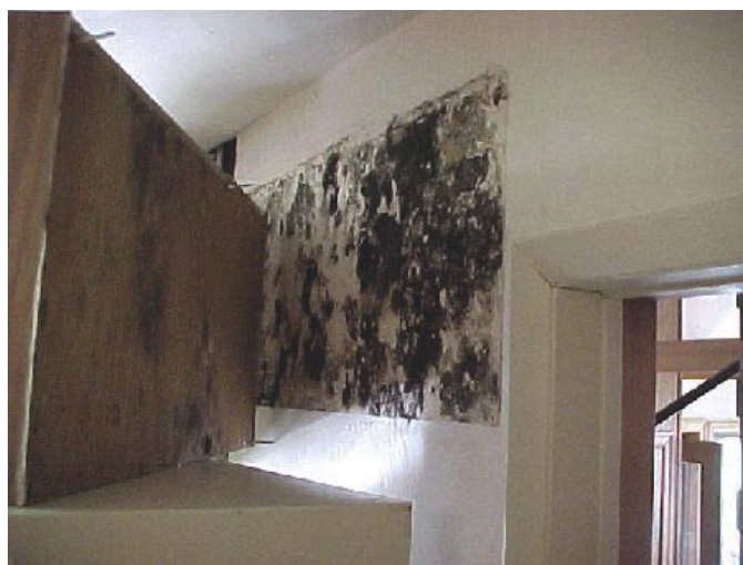
Figure 2. Some mold is hidden from view, such as the mold shown in this image, which was discovered when cabinets were removed from a wall (Photo courtesy of Mike McNickle)
