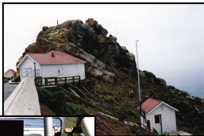
Figure 1. The measurement station (small building, right) at Point Reyes lighthouse, Northern California.
