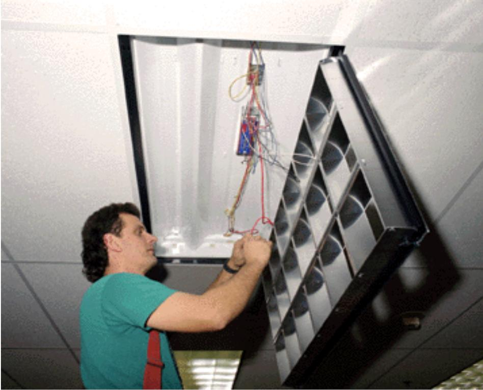
Figure 2: A contractor installs a dimming electronic ballast in a three-lamp lighting fixture at the Federal Building.
